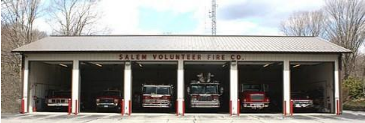
Figure 2. Salem Volunteer Fire Company Station, 424 Hartford Road (building owned by the town)
